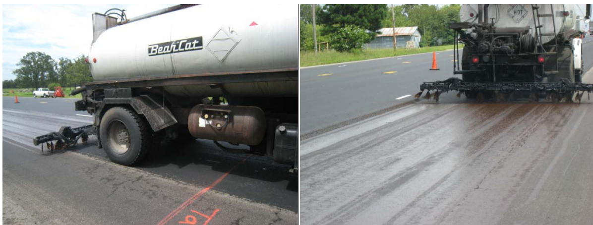
FIGURE 29 Tack Coat (SS-1) Applied by Contractor.
